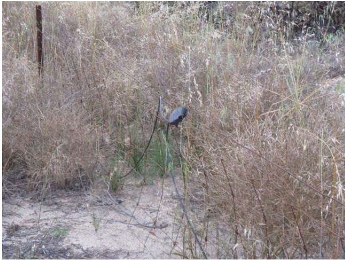
Photo 3. The cable join
