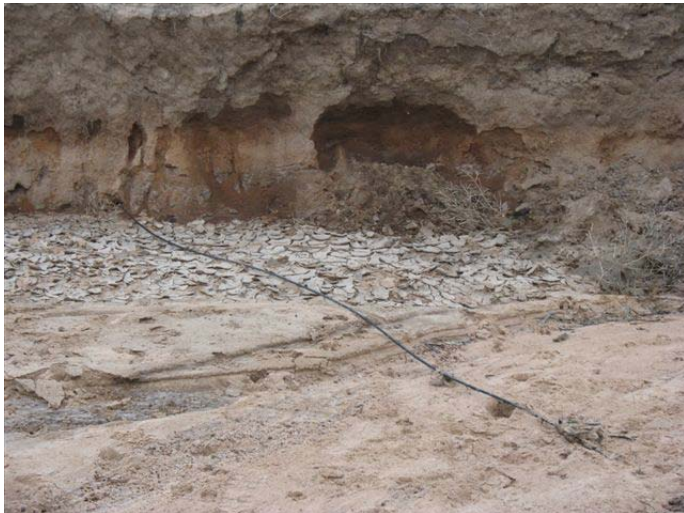
Photo 4. Cable lays across creek crossing - water flows from left to right.
