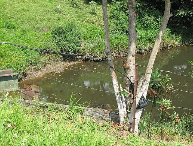
The phone cable connector in a plastic bag, duct taped to a fig tree near Green Bridge Stoney Chute.
